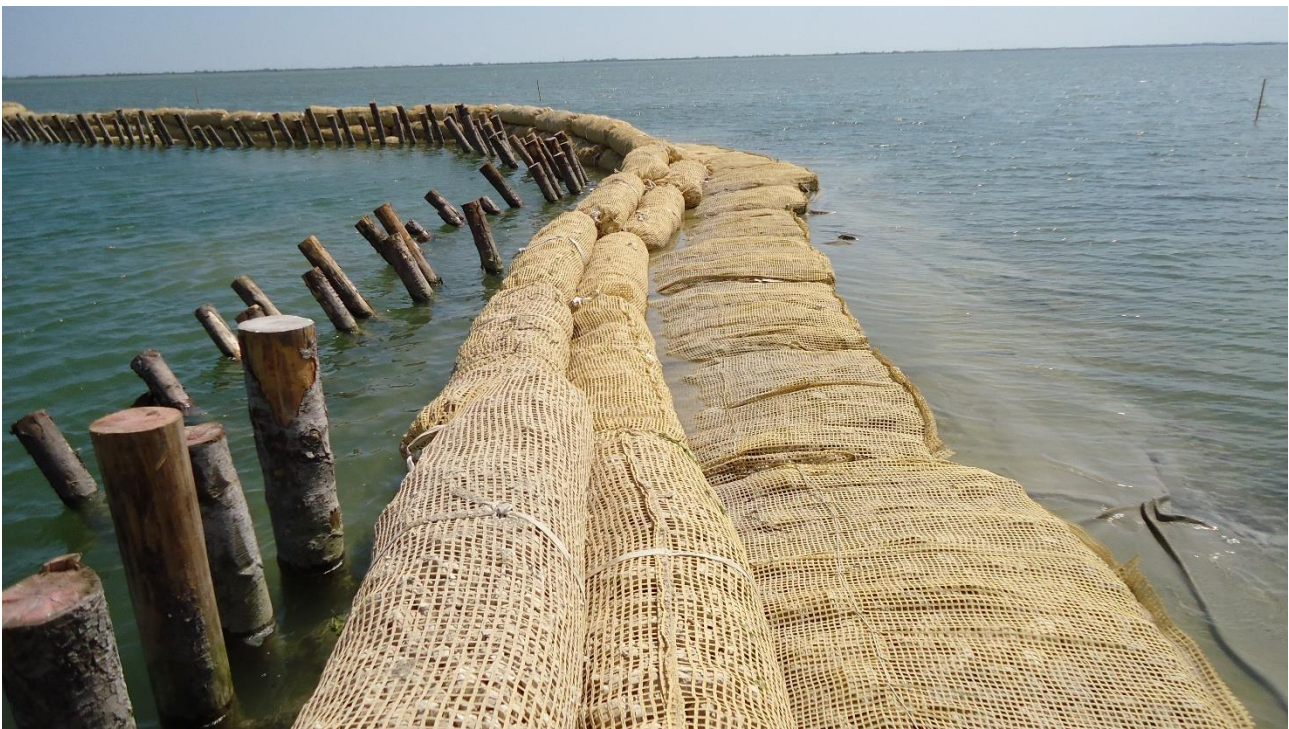
Figure 8.18 – Examples of implemented structures ( https://coedmar.it/portfolio-item/barena-ripristino-morfologico-area-canali-cenesa-boer-siletto/ ).
